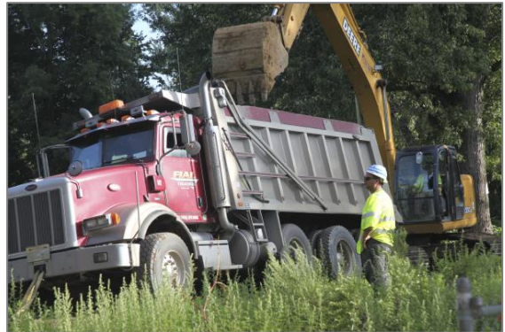
Debris removal operations in Lawrenceville, on September 9, 2011.
