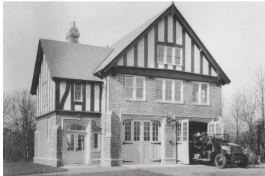
The New Fire Headquarters built in 1929. This building with major additions and renovations, is still Fire Headquarters today.
